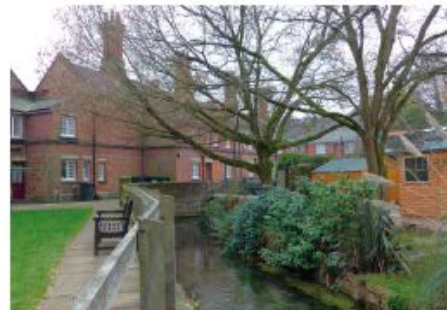
St John’s Almshouses boundary wall
